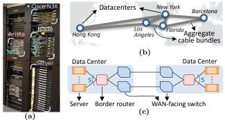
Figure 8: Our testbed. (a) Partial view of the equipment. (b) Emulated DC-level topology. (c) Closer look at physical connectivity for a pair of DC.
